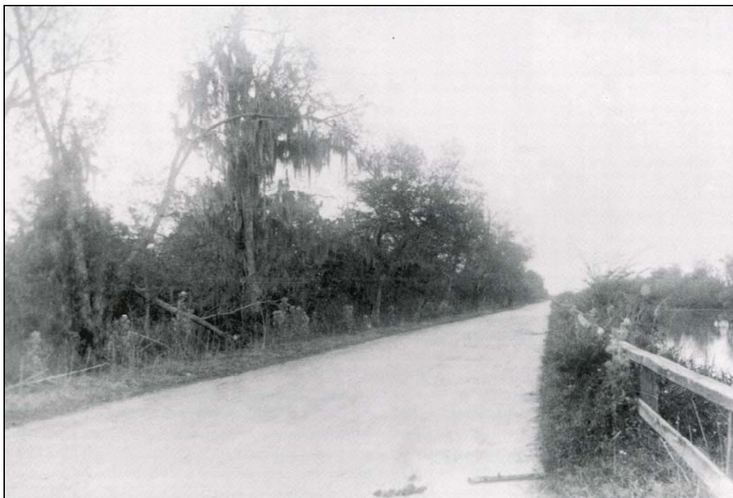
Figure 4.18 – Photo taken in 1890 looking north along the “shell road” than ran along the west side of the New Basin Canal, seen at extreme right. Note the modest height of the original embankment, no more than 5 feet above the adjacent cypress swamp at left. The original embankments were heightened after hurricane-induced overtopping in 1915 and 1947 (image from the University of New Orleans Special Collections, New Orleans Views).
