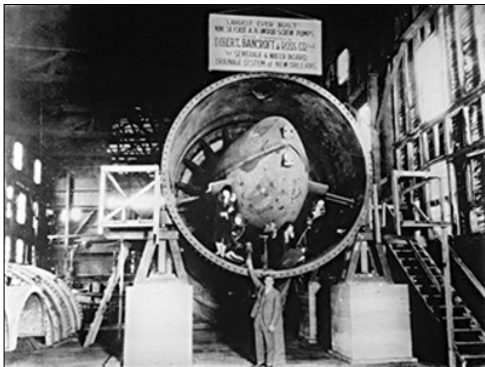
Figure 4.21: S&WB engineer A. Baldwin Wood standing next to one of his 14-foot diameter screw pumps in 1929 with several of the board's secretaries sitting inside the housing for scale (courtesy of the Sewerage & Water Board of New Orleans).
