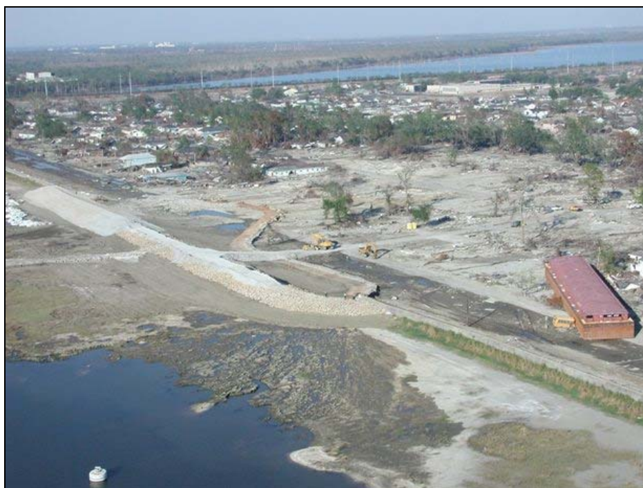
Figure 4.31: Seepage crevasse splay exposed on the water side of the east levee of the IHNC breach after Hurricanes Katrina and Rita. This same section of the IHNC levee failed in 1965 during Hurricane Betsy. Levees tend to fail during sustained high flow events because of underseepage problems, toe scour, and overtopping. Note the anomalous seepage in lower foreground, which suggests much higher permeability in this particular portion of the dike, close to the south end of the failed section (photo from Army Corps of Engineers).
